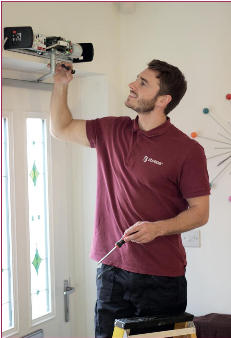
Steeper Engineer, Jon installing an automatic swing door opener.
